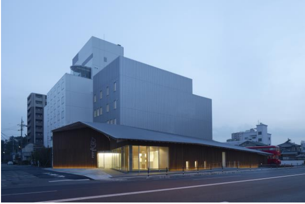
HOSPITAL HIKARI, JAPAN KENGO KUMA & ASSOCIATES
